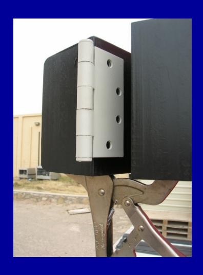
Hinge aligned with mounting pins ready to close. Use caution when closing to avoid pinching hand
