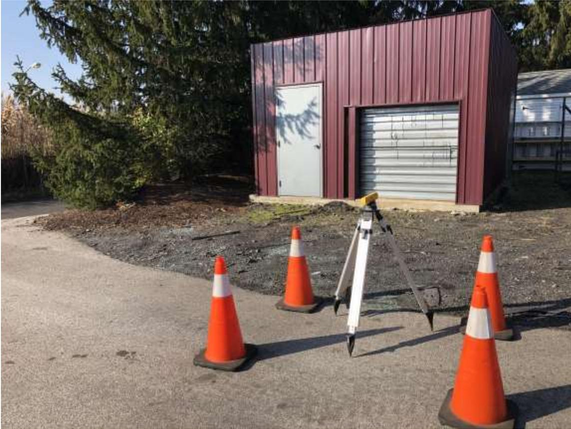
Above – Tripod and Laser set up is established on a firm base with cones to prevent accidental knocking or movement of the equipment.
